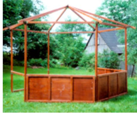
**1.** Start assembling the frame with the **corner posts** and **side panels**. First use two side panels to support the frame. Try not to twist the connector hinges, they might otherwise get blocked. Make sure the **side panels** are in the correct orientation, some might have hinges for the counter.
